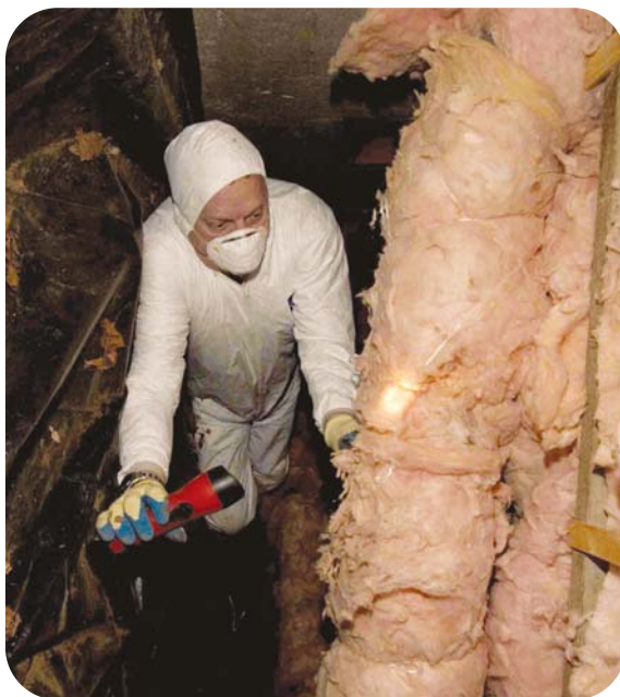
Rod Street, Home Performance with Energy Star account manager for CSG, examines a home's insulation.
